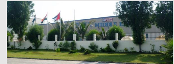
Flex Films (UAE) state-of-art facility has an installed capacity to produce over 22,000 MT of BOPET Films per annum
