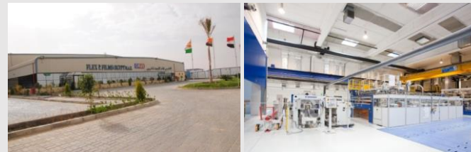
Flex Films (Egypt) state-of-art facility has an installed capacity to produce over 1,14,000 MT of BOPET/BOPP/ CPP Films p.a.
